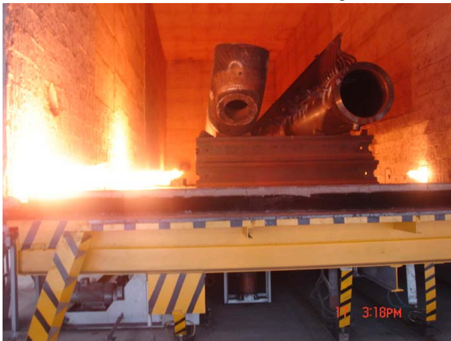
Heat Treatment furnace where the Super Heater Coils were placed
